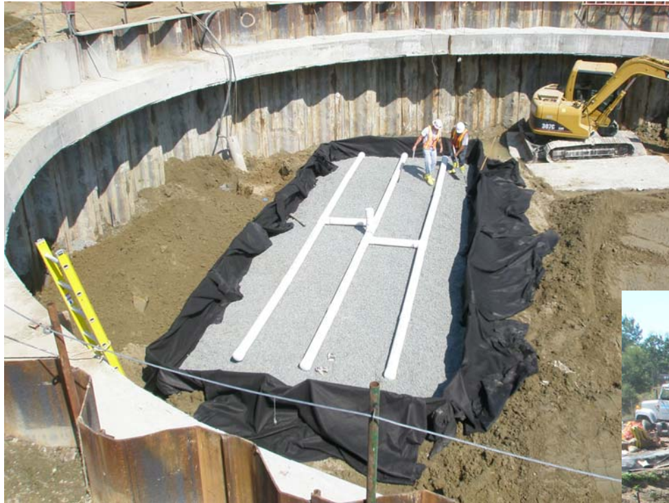
Installation of Infiltration Gallery in Western Portion of Excavation
