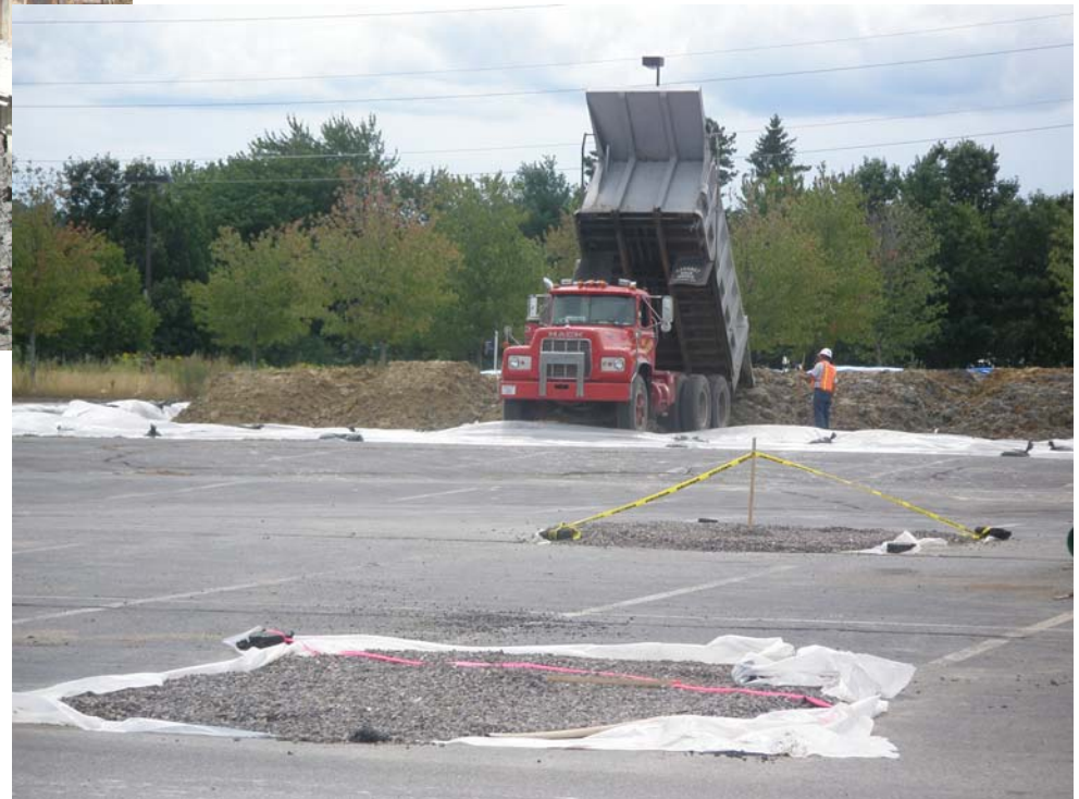
Transportation of Soil to Staging Area in Parking Lot
