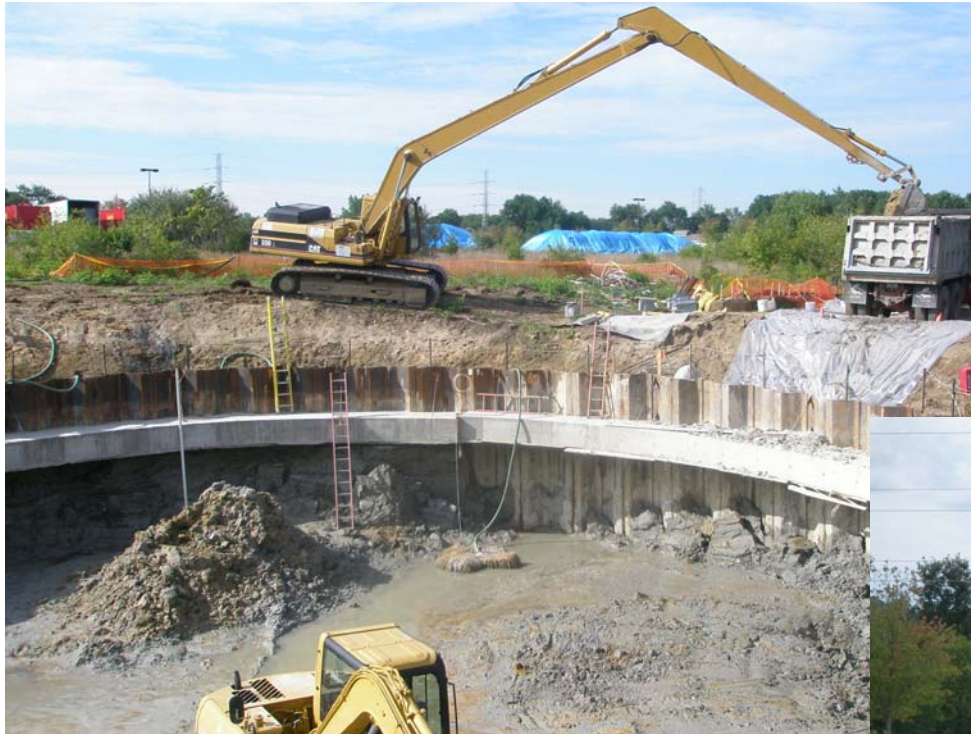
Transportation of Soil from Excavation
