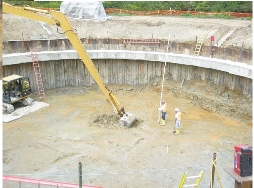
Excavation of Potholes
