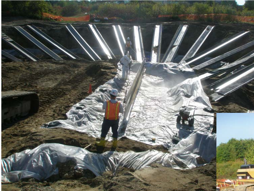
Sheet Pile Decontamination
