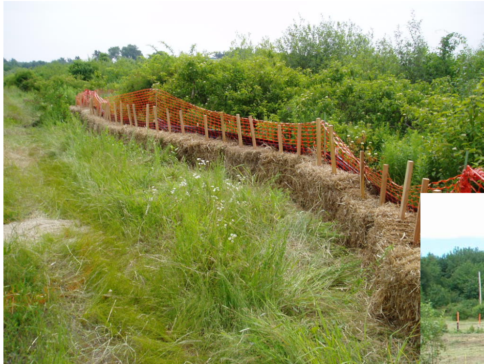
Silt Fence with Straw Bales and Construction Fence
