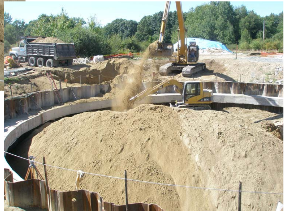
Backfilling Excavation
