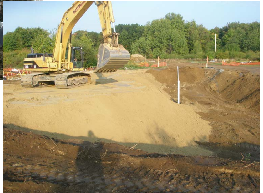
Backfilling Excavation
