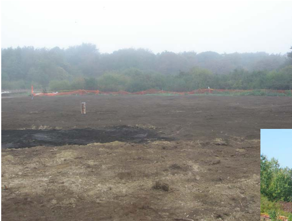
Completed Excavation Area Grading
