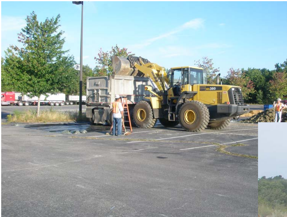
Loading Trucks for Off-Site Disposal
