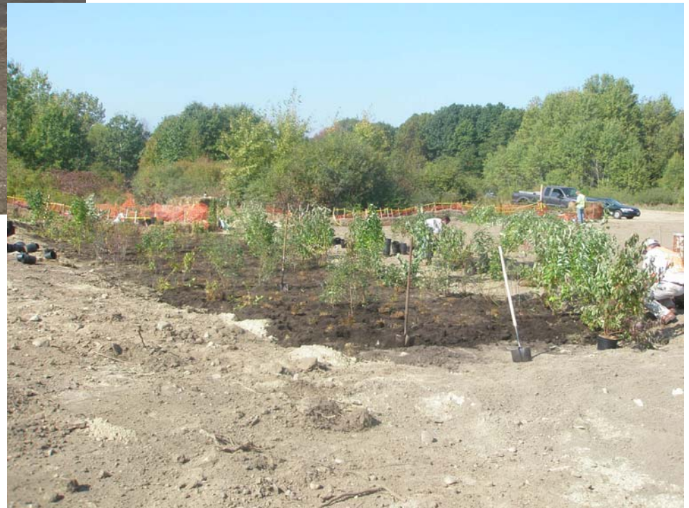
Completed Wetland Restoration
