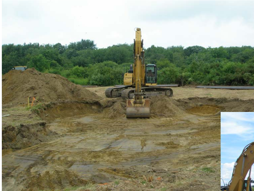
Excavation of Cofferdam Area
