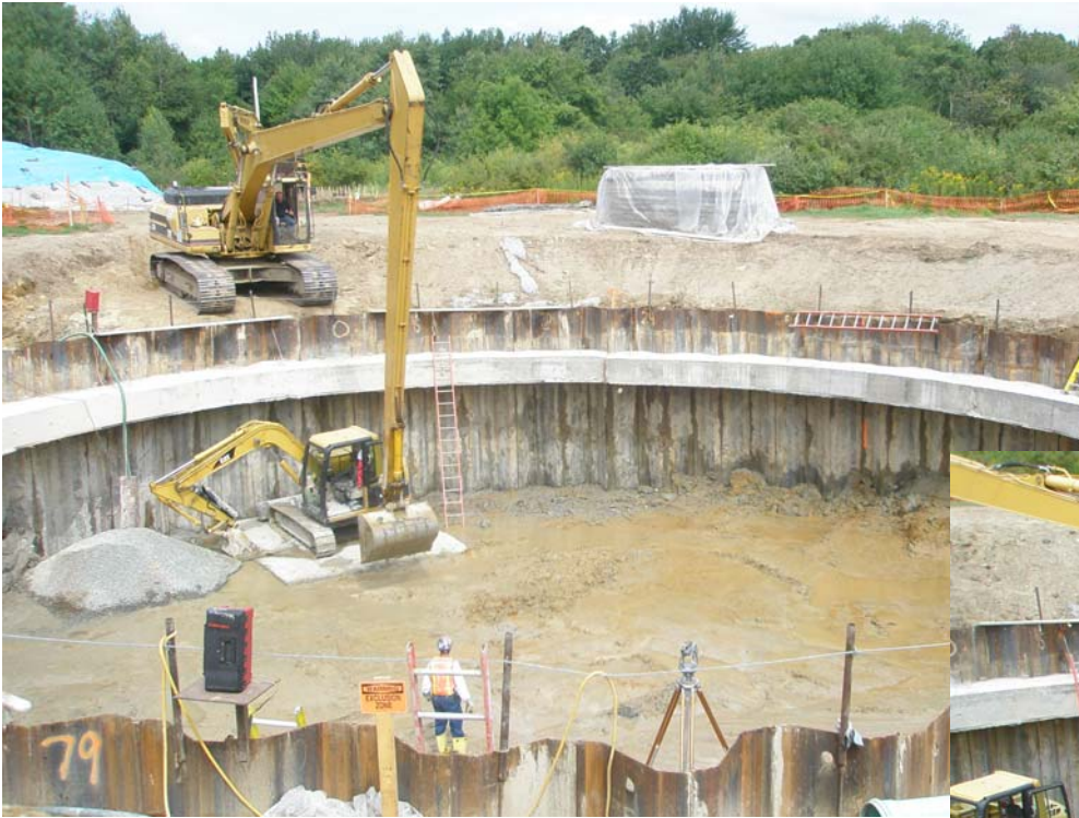
Maximum Depth of Excavation
